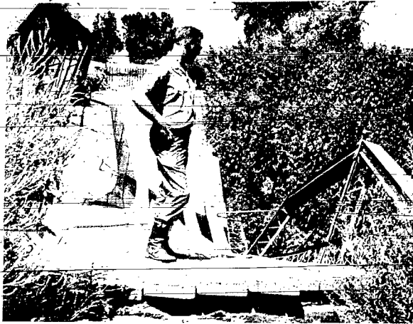
Bob Nissen, county road superintendent, checks over a bridge three miles west and about a quarter mile north of Wayne. The bridge was damaged earlier this summer when a car hit the railing. Cost of replacing the bridge is estimated at near $20,000.
